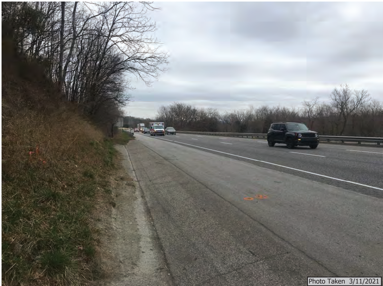
8. Facing east along I-64, west of I-265 interchange
