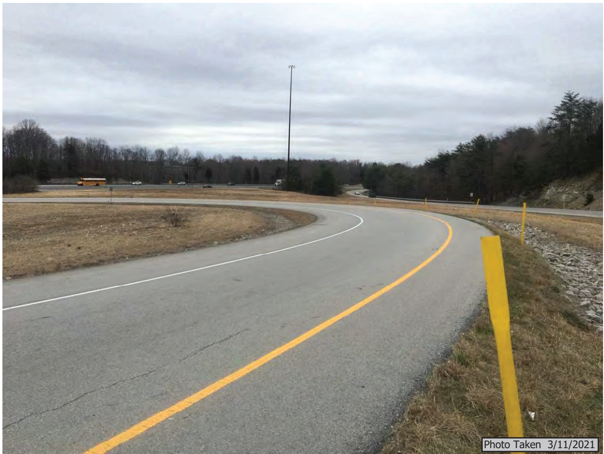
1. Facing northeast at I-64 and US 150 interchange
