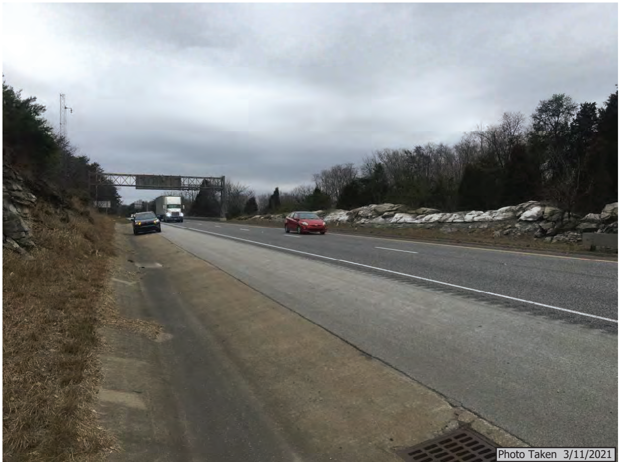
6. Facing northwest on I-64, east of US 150 interchange
