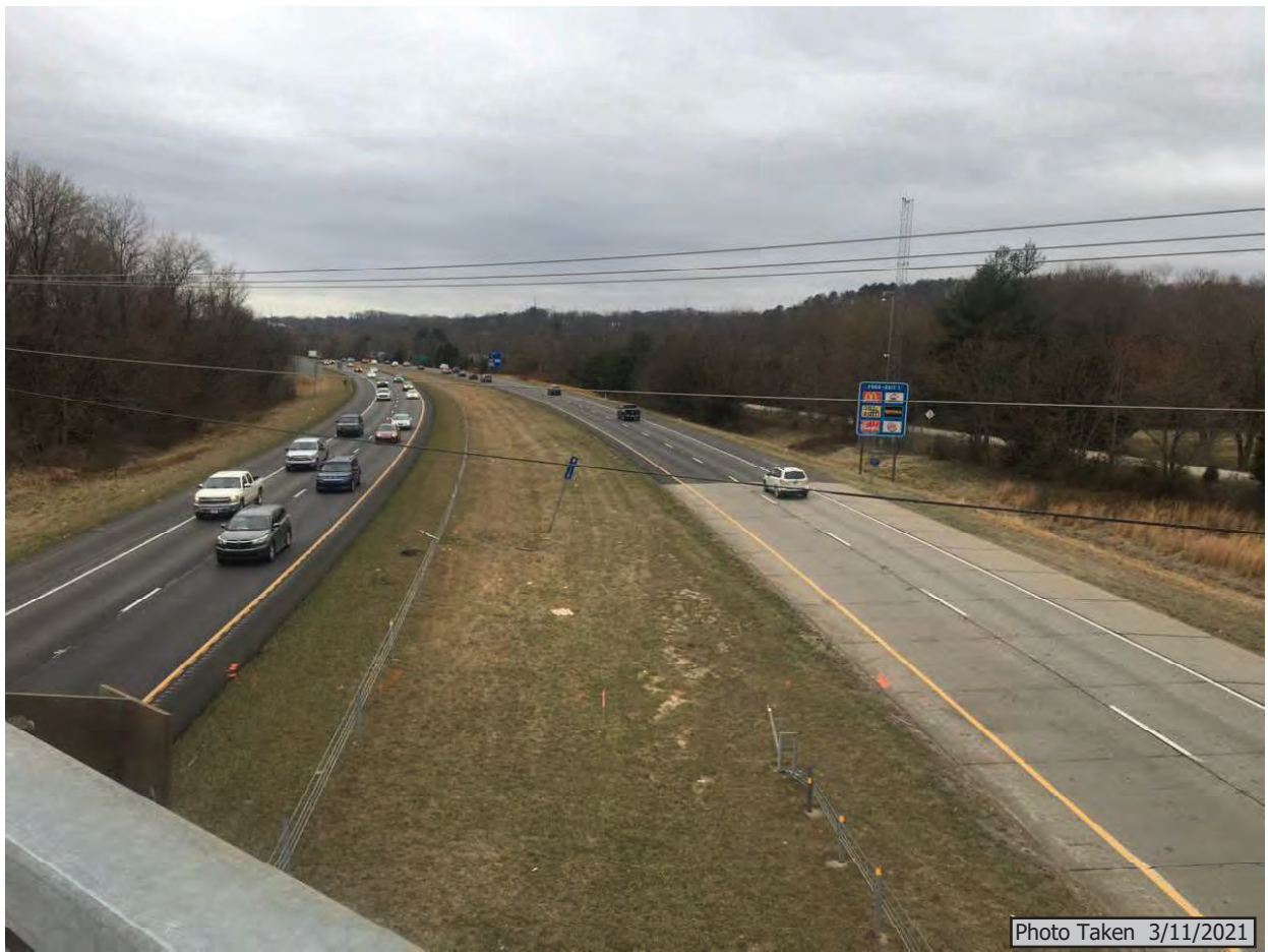
21. Facing southwest to I-265 from Green Valley Road overpass
