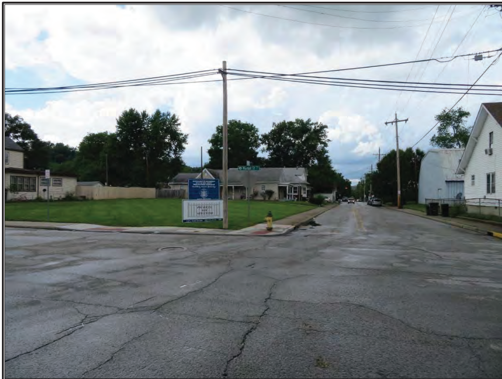
Figure B-18. Overview of the West End Historic District at the intersection of Market Street and West 7th Street, facing northwest.
