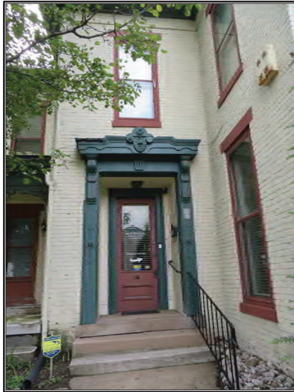
Figure 43. Detail of the east elevation of the Reyse (Roy[s]ce)-Friend House (IHSSI 043-446-34204), facing southwest.
