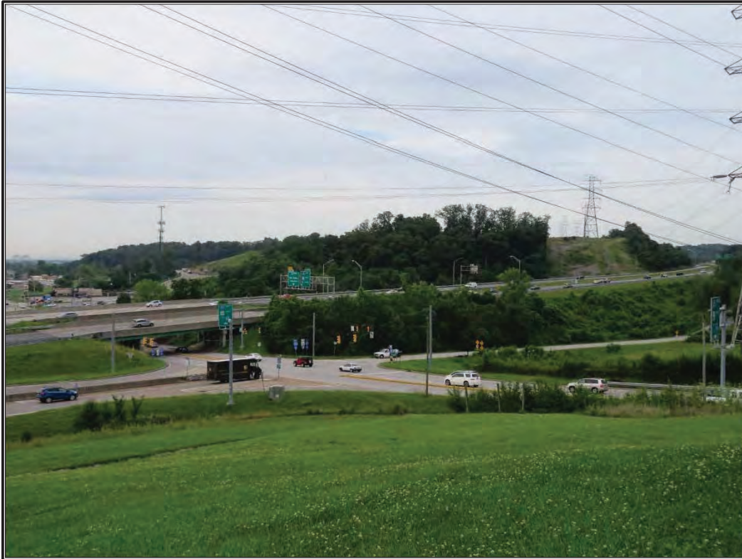
Figure 3. Overview of project area and APE from Paoli Pike Road, facing southeast.
