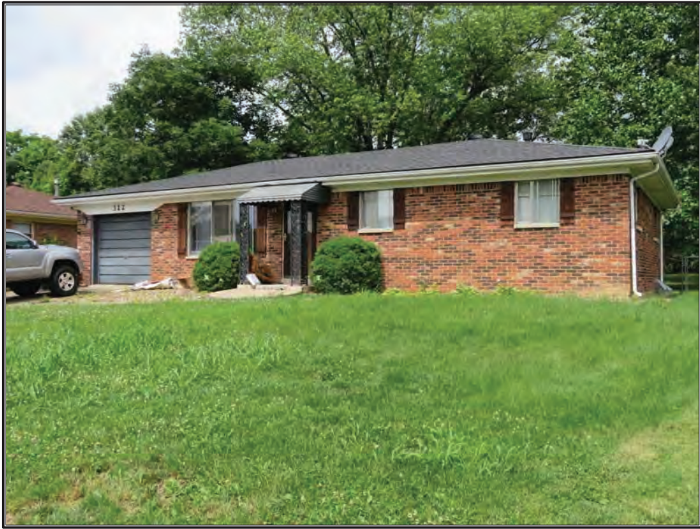
Figure 12. View of INDOT 47, facing southeast.
