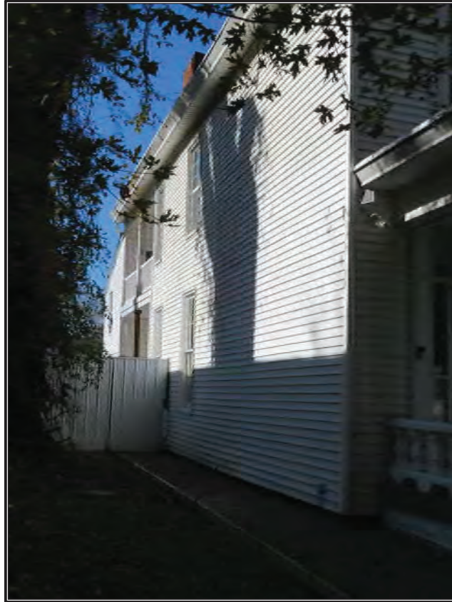
Figure 32. South elevation of House (IHSSI No. 043-446-34245), facing west.
