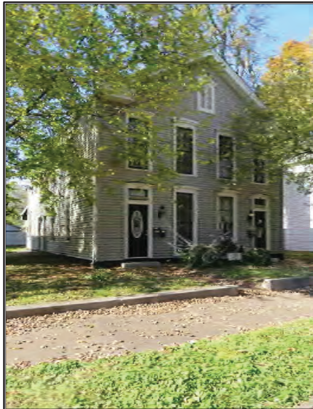
Figure 25. Façade (east) and south elevation of House (IHSSI No. 043-446-34246), facing southwest.
