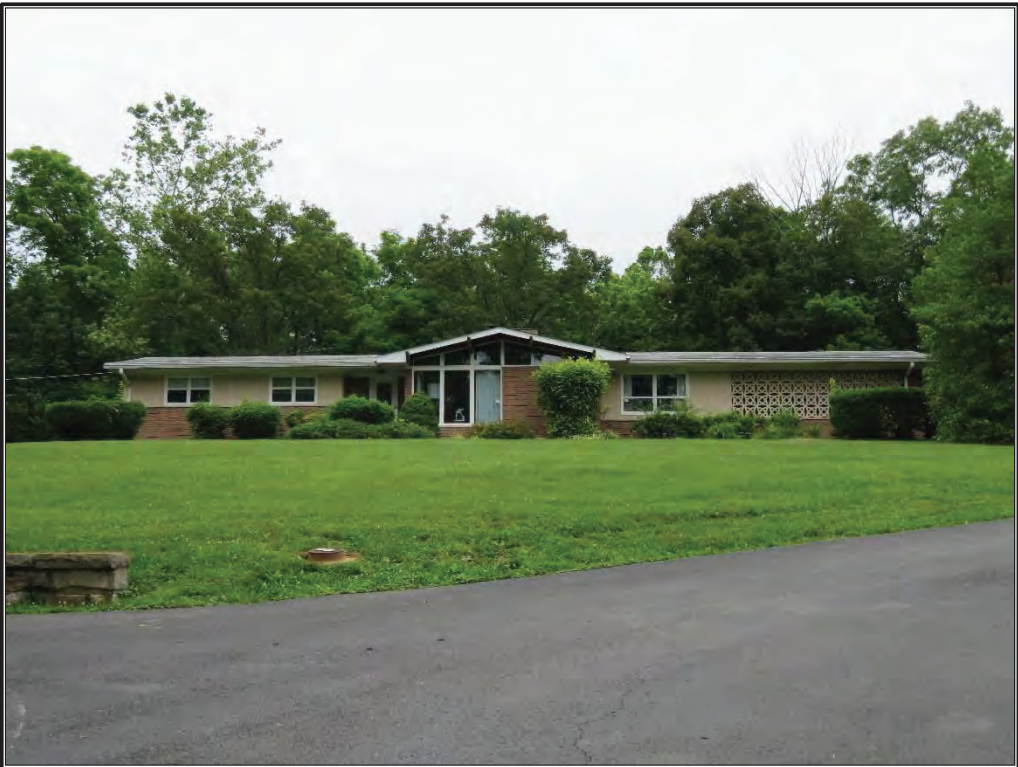
Figure 17. View of INDOT 23, facing northeast.
