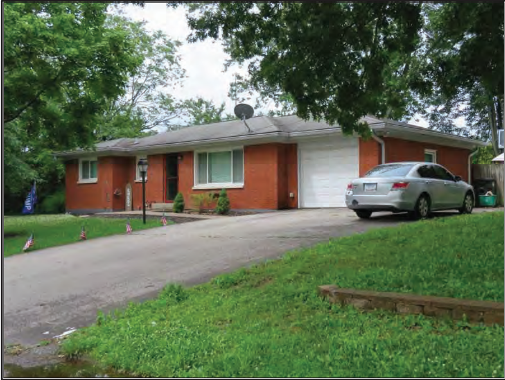
Figure 6. View of INDOT 73, facing southwest.
