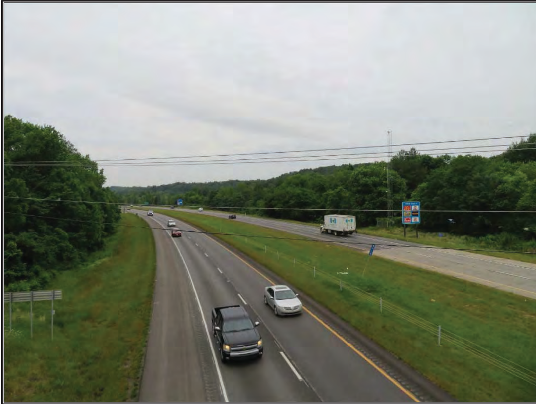
Figure 2. Overview of project area at the Green Valley Road bridge overpass over I-265, facing southwest.
