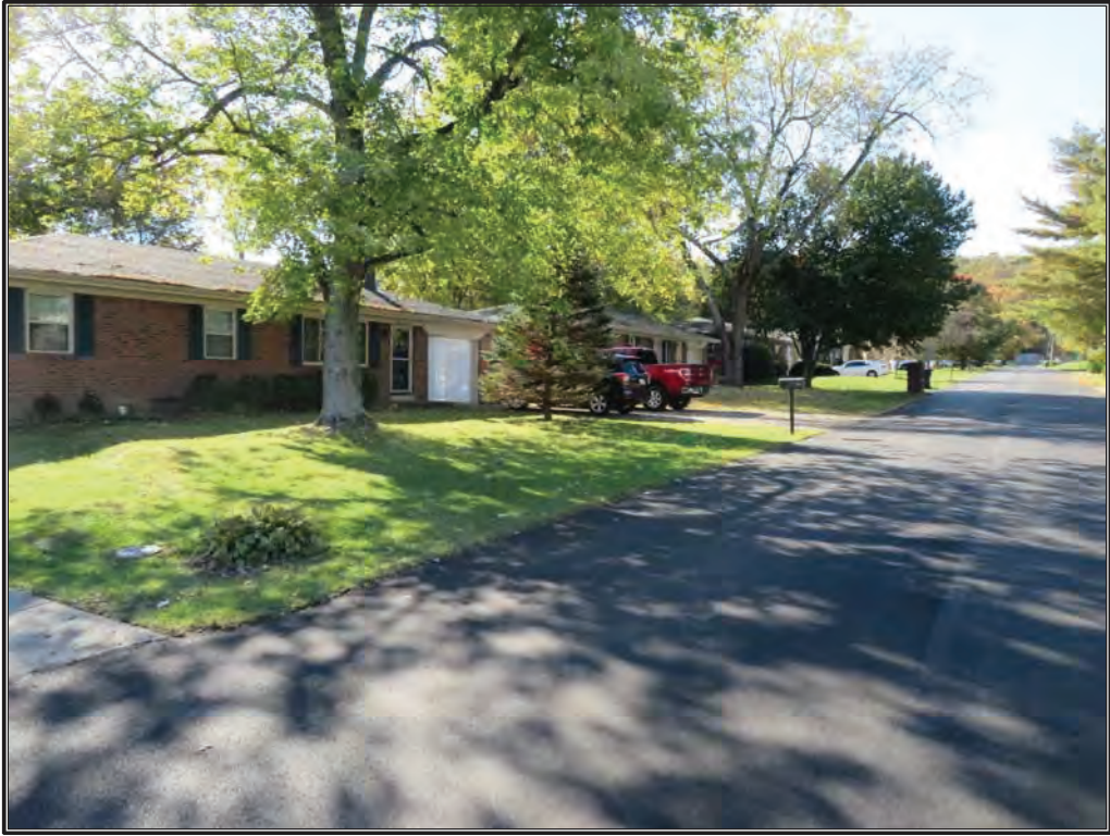
Figure 22. Overview of Village Pines Subdivision, facing southeast.
