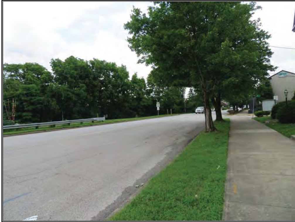
Figure B-7. Overview of the project area and the APE at the intersection of along East Spring Street, near the James Carr House and Reyse (Roy[s]ce)-Friend House, facing northeast.
