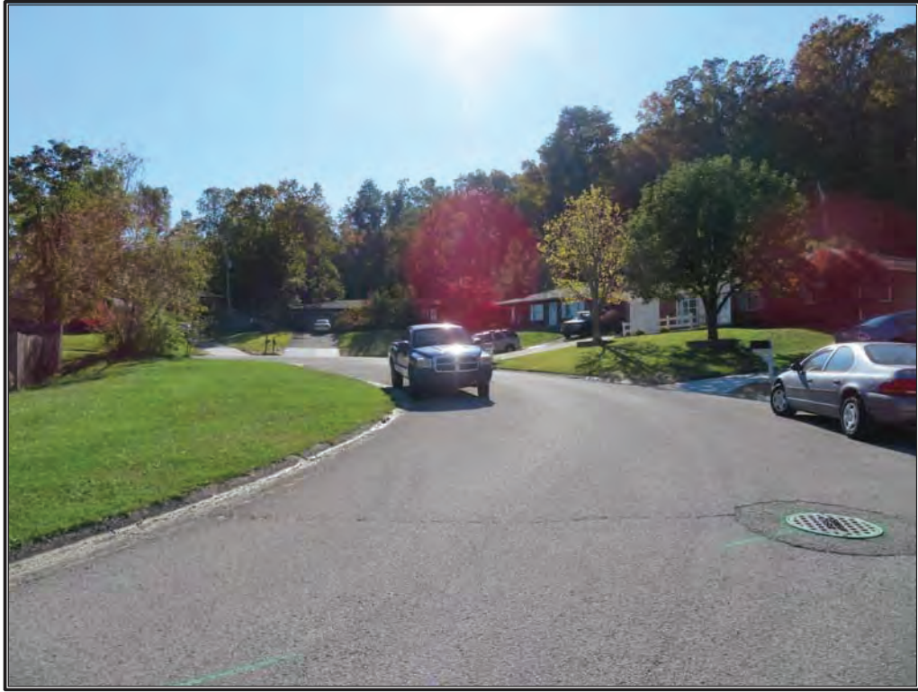
Figure 23. Overview of Village Pines Subdivision, facing southwest.
