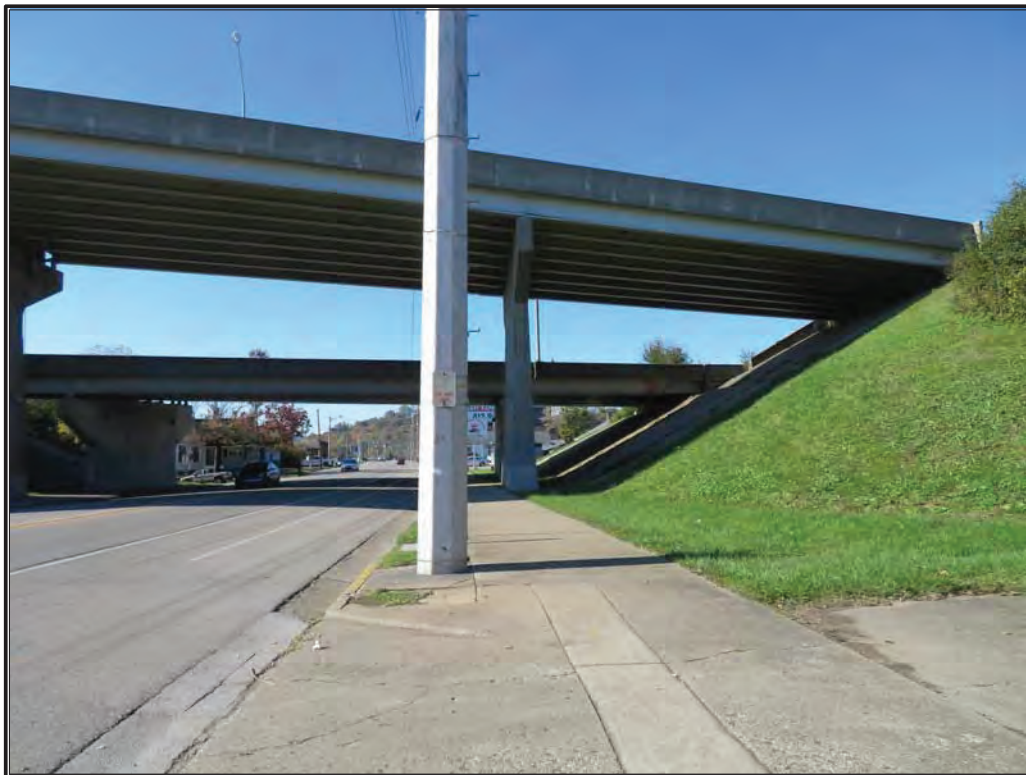
Figure B-26. Overview of the project area along West Main Street, facing west.
