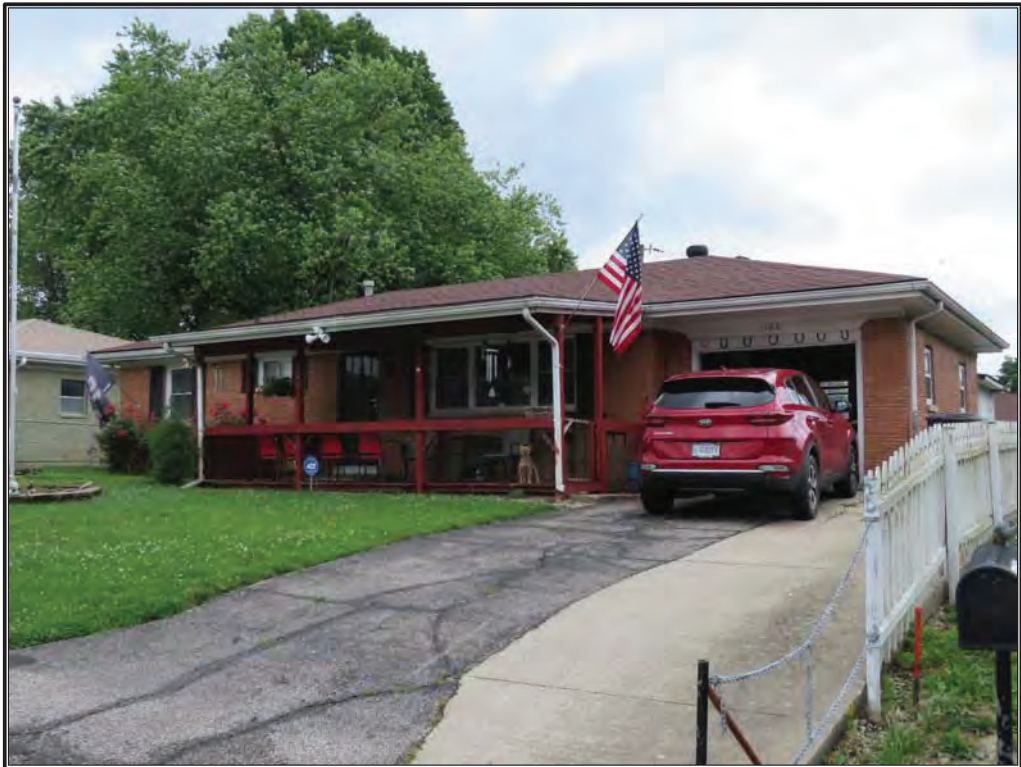
Figure 7. View of INDOT 58, facing northeast.
