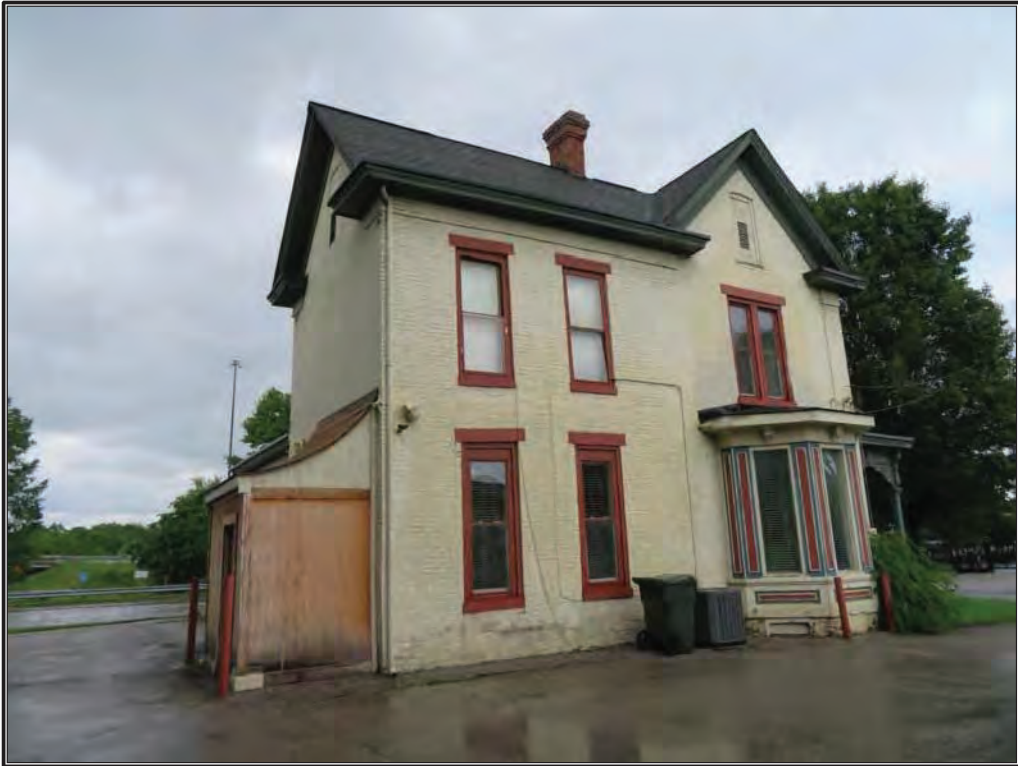
Figure 45. Rear (south) and west elevation of the Reyse (Roy[s]ce)-Friend House (IHSSI 043-446-34204), facing south.
