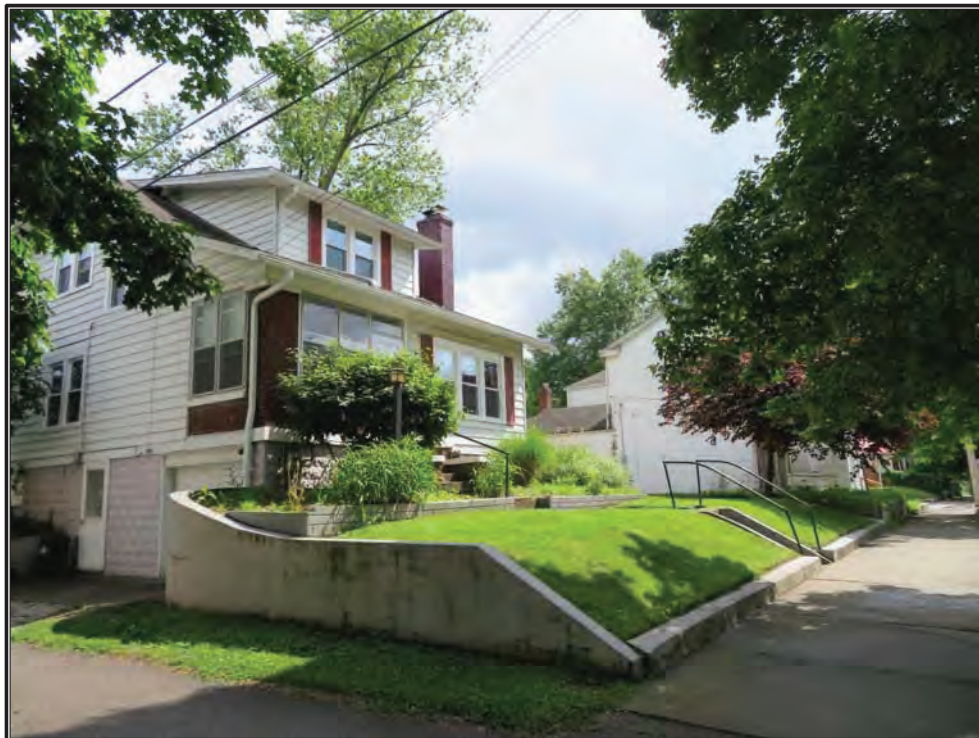
Figure B-22. Overview of the West End Historic District along West Spring Street, facing southwest.
