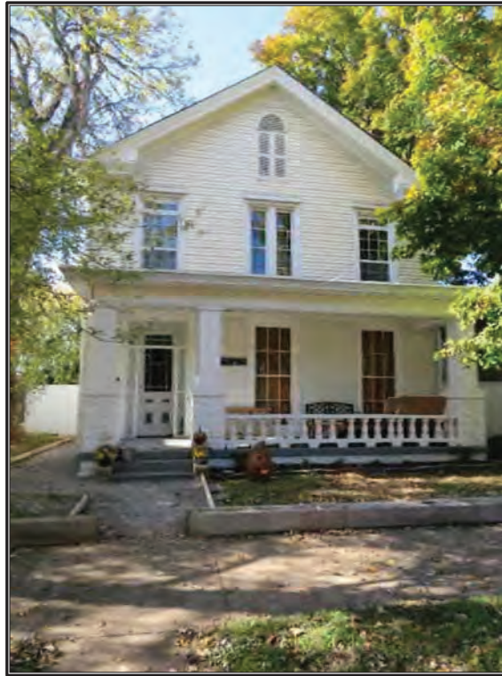
Figure 30. Façade (east) elevation of House (IHSSI No. 043-446-34245), facing southwest.
