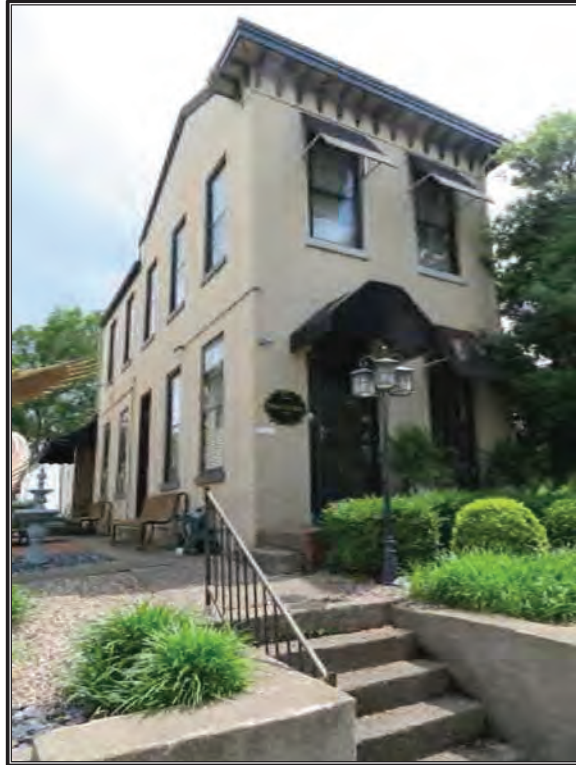
Figure 35. Façade (north) and east elevation of the James Carr House (IHSSI No. 043-446-34202), facing south.
