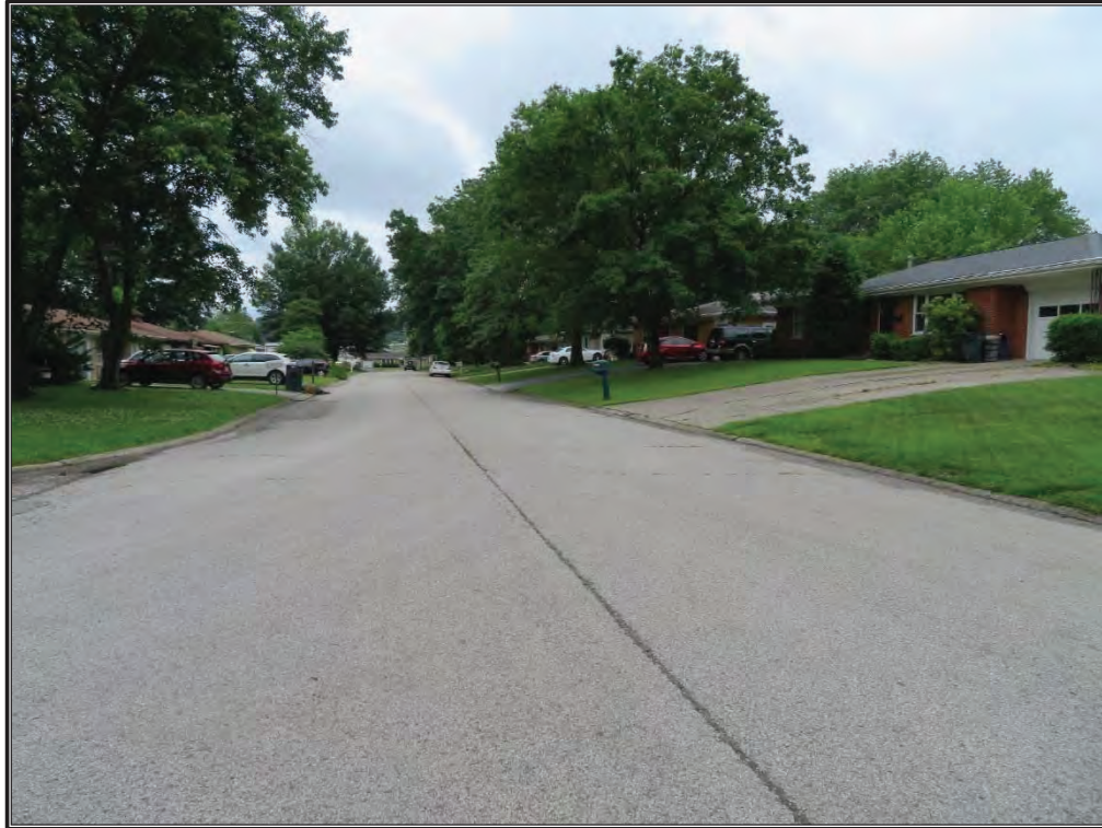
Figure B-15. Overview of 1950s and 1960s residences associated with the Finchland Subdivision along Rossmore Drive, facing southwest.
