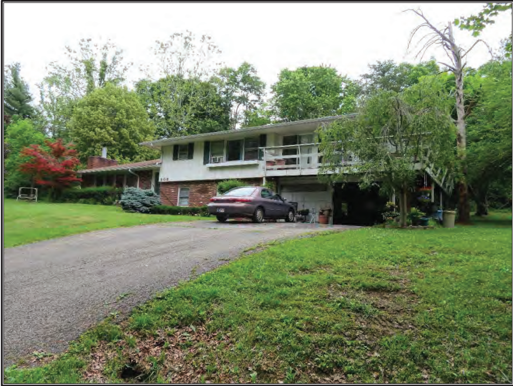
Figure 16. View of INDOT 22, facing northwest.
