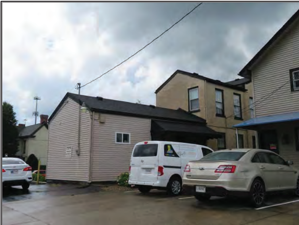
Figure 37. Rear (south) and east elevation of the James Carr House (IHSSI No. 043-466-34202), facing west.
