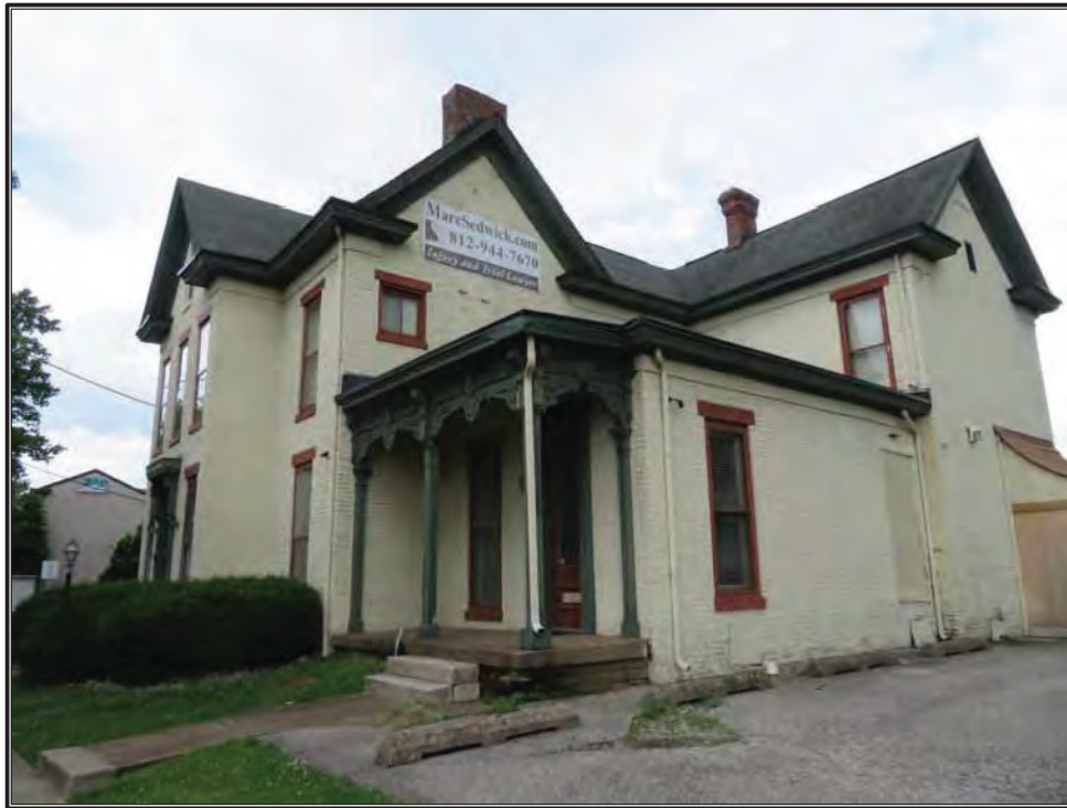
Figure 41. Façade (north) and west elevation of the Reyse (Roy[s]ce)-Friend House (IHSSI 043-446-34204), facing east.
