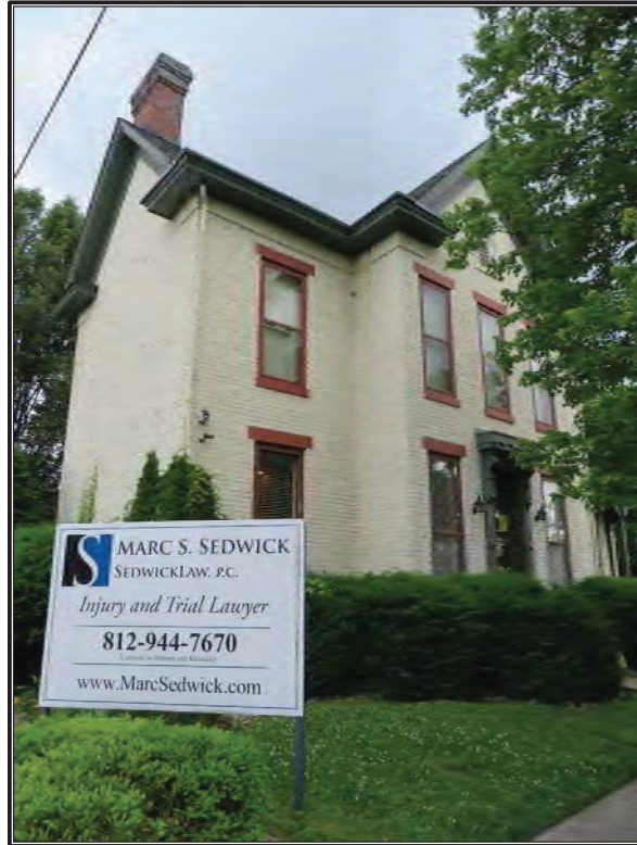
Figure 39. Façade (north) and east elevation of the Reyse (Roy[s]ce)-Friend House (IHSSI 043-446-34204), facing south.
