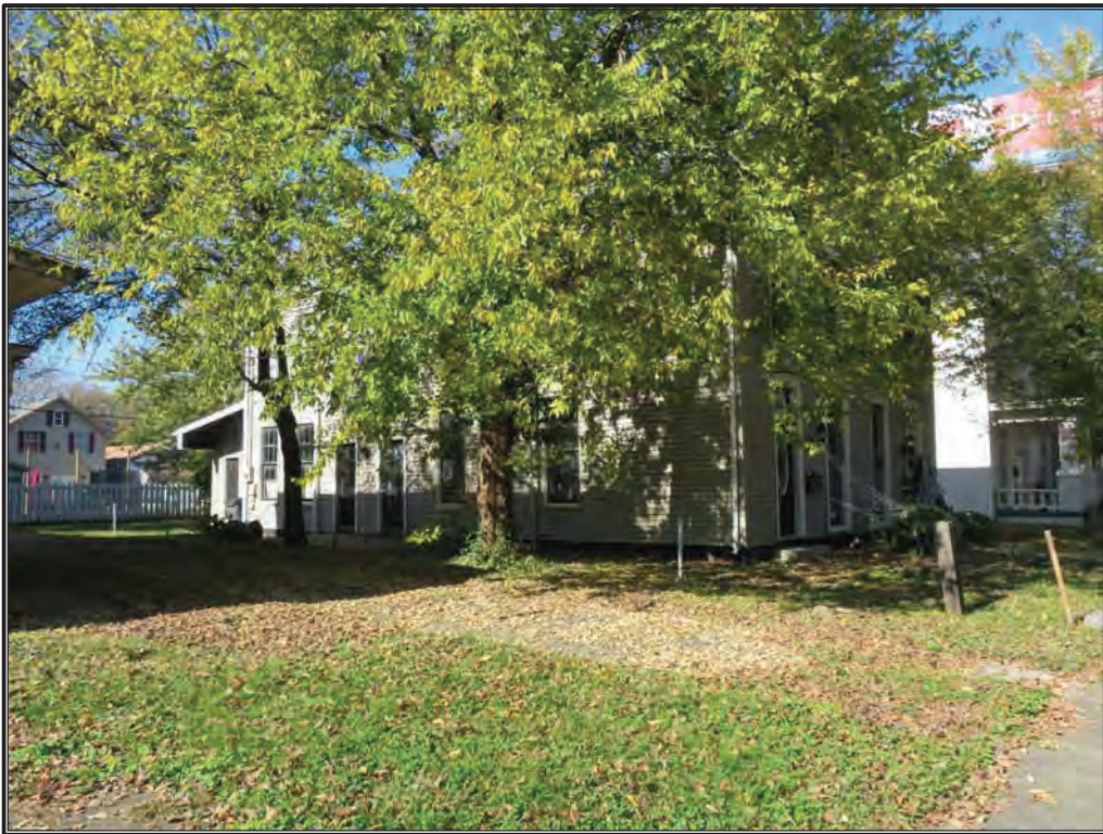
Figure 27. Façade (east) and south elevation of House (IHSSI No. 043-446-34246), facing west.
