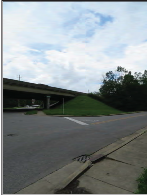
Figure B-5. Overview of the project area at the intersection of Cherry Street and West Street, facing northwest.
