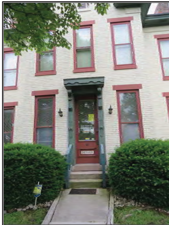
Figure 40. Detail of the façade (north) elevation of the Reyse (Roy[s]ce)-Friend House (IHSSI 043-446-34204), facing southeast.
