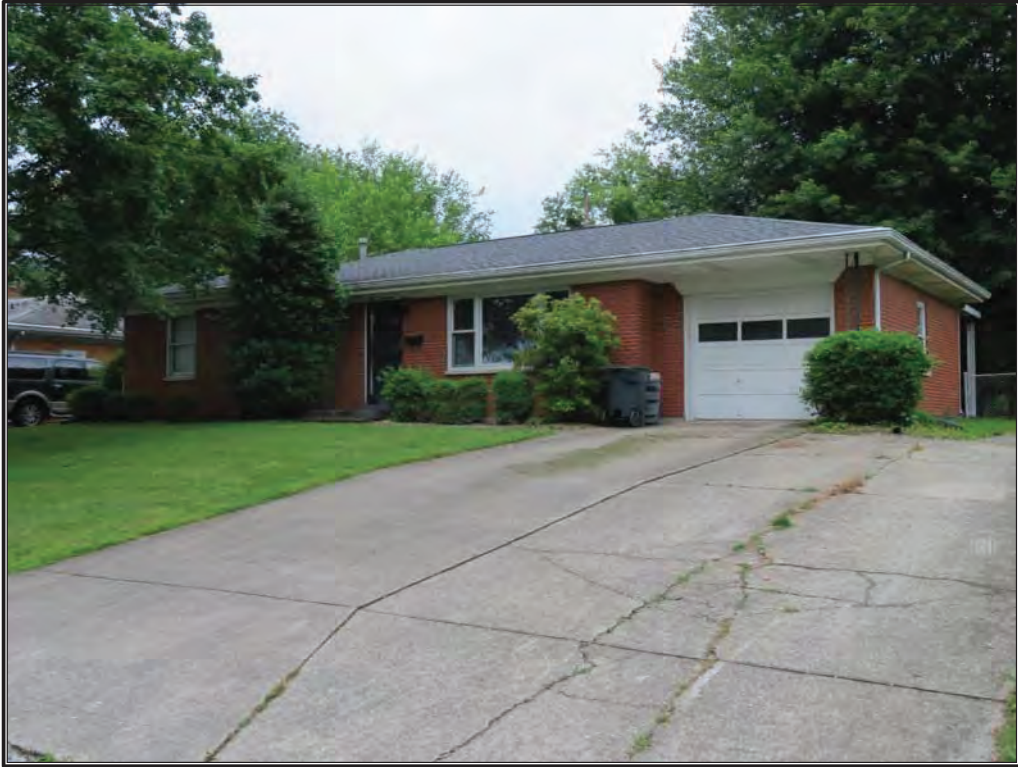
Figure 8. View of INDOT 66, facing southeast.
