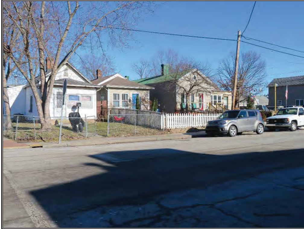
Figure B-8. Overview of the West End Historic District at the intersection of West Market Street and West 8th Street, facing north.
