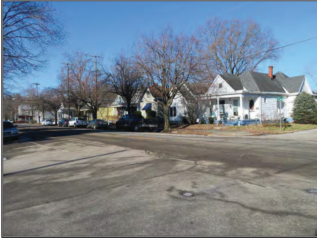
Figure B-2. Overview of the West End Historic District at the intersection of West Spring Street and West 6th Street, facing northwest.
