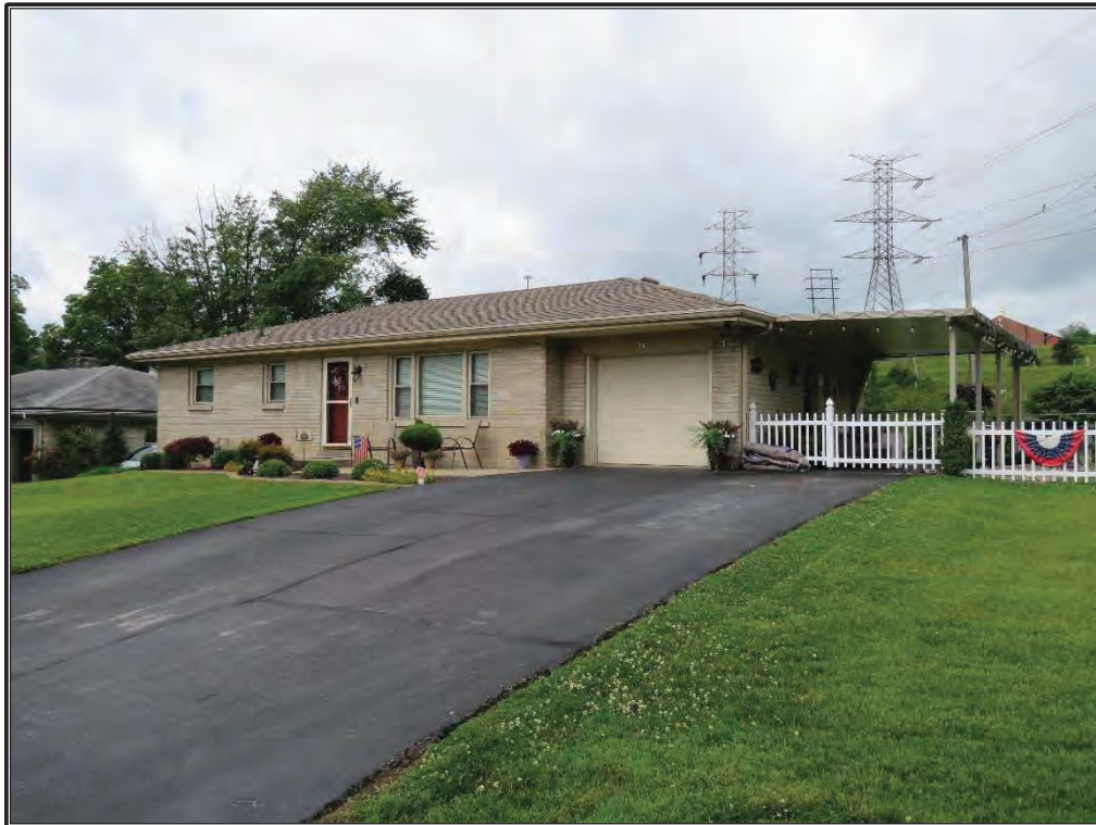
Figure B-13. INDOT 57 facade (east) and north elevation, facing southwest.
