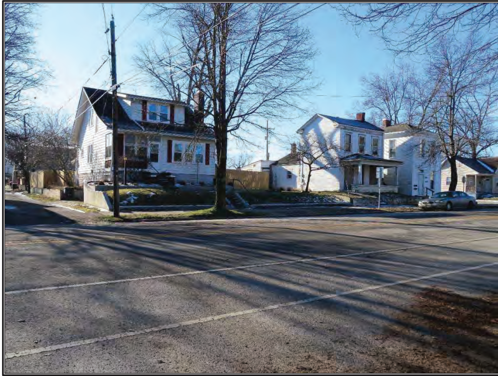
Figure 8. Overview of the West End Historic District along the south side of West Spring Street, facing southwest.
