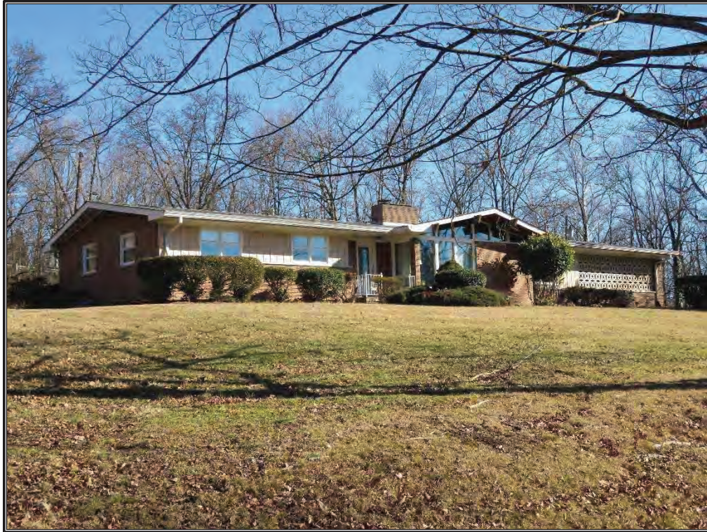
Figure 29. Facade (south) and west elevation of INDOT 23, facing northeast.
